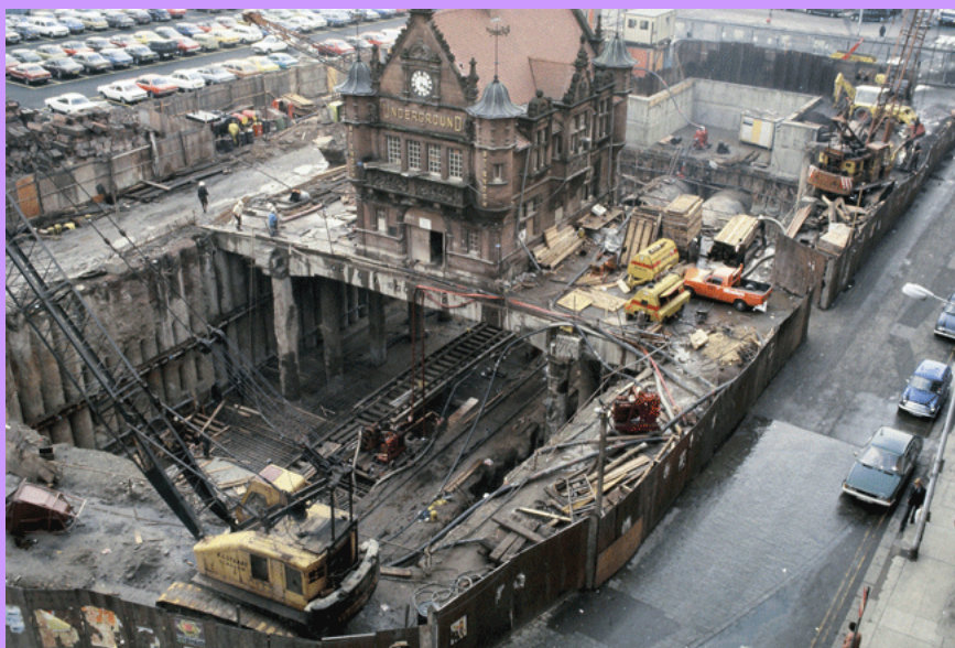
1977 Reconstruction found the original offices on pylons while work proceeded!
